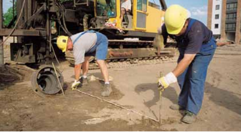
protection of the drill hole
